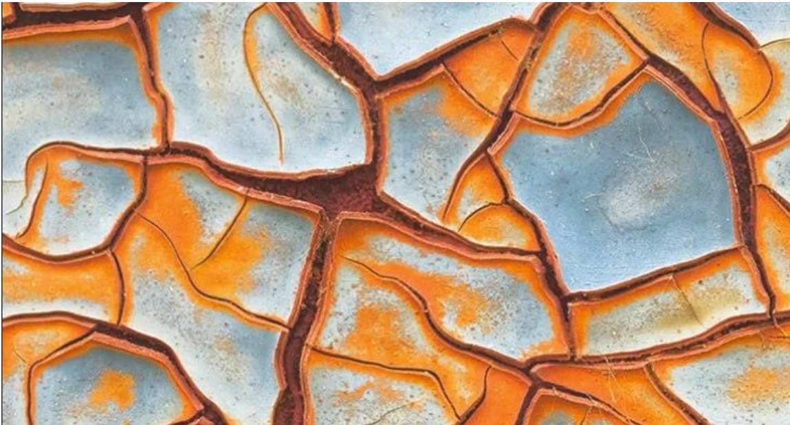
Figure 1: Sample Crack Pattern.
