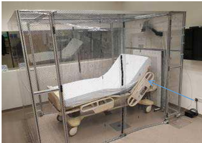
Fig 2: The Negative Pressure Full Isolation Tent over the Bed (the arrow represents the HEPA filter)
